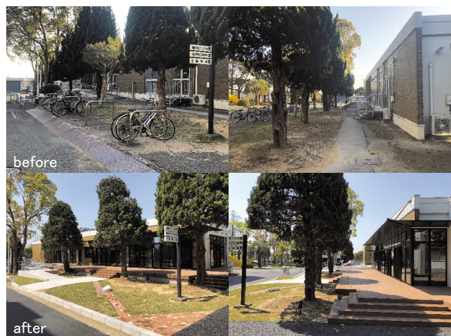
Fig.12 Before/after of east exterior
