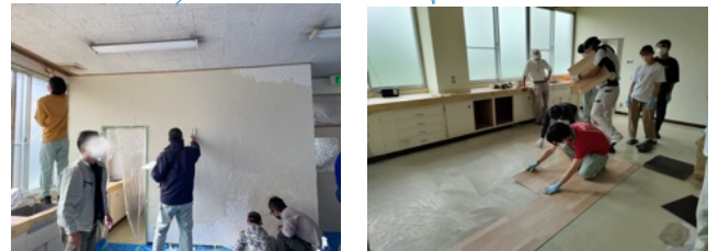
Fig.3 Renovate areas and working scenes
